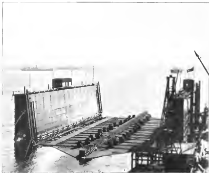
Above—View of the deck of the starboard wing of the smaller section of dock showing one of the four flood gate valve operating stands, one of the four flapper valve operating stands, the motor house, and the horizontal line shafting driving the pumps. The graduated spars are the water gauges for the pontoon. At right—View looking down on the small section of the dock showing the general arrangement.
